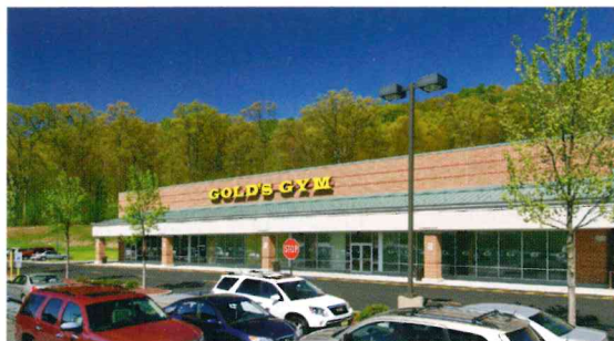
Gold's Gym, Flanders, N.J. - The new 15,000-square-foot structure was built by Klae for the landlord. The fit-up work was completed for Gold's Gym's owner.
