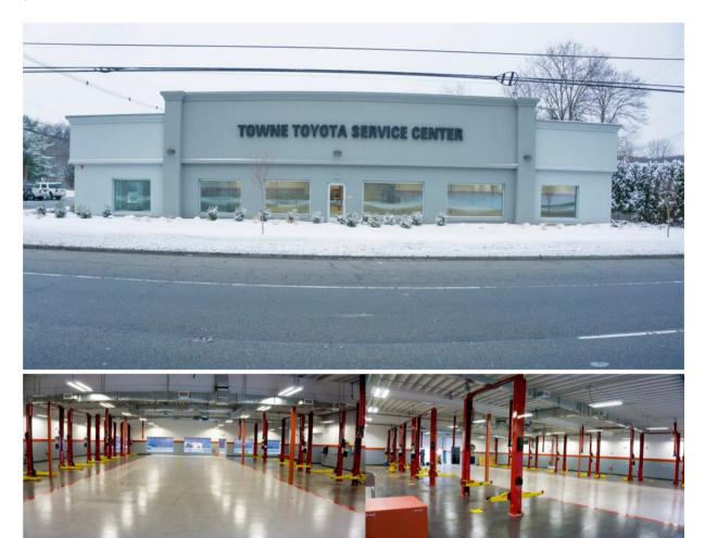
This project was a renovation of an existing one-story building for Toyota's new Service Center. Klae Construction raised the existing roof structure to accommodate the height requirements for new auto lifts.
