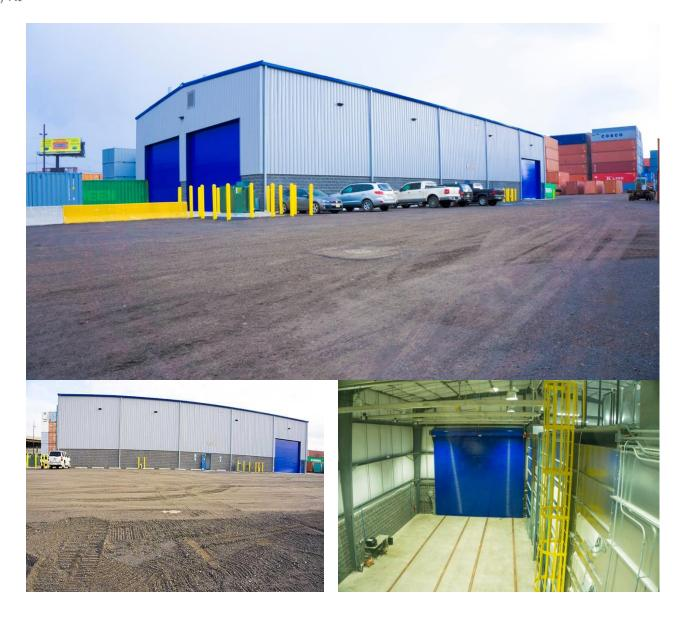
Klae Construction completed a 12,000 ft<sup>2</sup> pre-engineered steel building for Interport in Newark, NJ. This steel building shop-facility included a 1,100 ft<sup>2</sup> mezzanine. The construction also included an existing building demolition and site utility installations.
