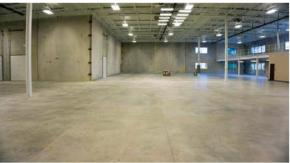
After the roof collapsed and severely damaged the previous structure, Klae Construction reconstructed the 20,500 ft2 building. The reconstruction included new footings and concrete slabs; tilt-up concrete walls; structural steel columns with bar joist and steel roof deck; new equipment mezzanine; loading docks; complete building sprinkler system; new electric service and lighting; and new administrative offices, break room, conference room, and restrooms.
