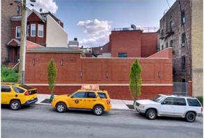
Klae Construction completed this addition for the Franciscan Sisters of St. Elizabeth in Jersey City. The 4,700 ft2 addition includes a playground with a parking garage below it. The new parking garage is fully heated with a directional lighting system to control traffic flow. An elevator was constructed to link the playground to the existing structure. The playground was built from the ground up and contains stairwells, a handicap
