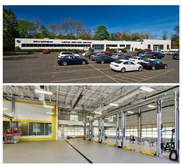
KLAE CONSTRUCTION COMPLETED THIS ADDITION to the Ray Catena MINI Cooper service center on Yellowstone Avenue in Greenburgh, NY. The 7,000 square-foot building addition with structural steel frame and concrete block walls includes a 1,200 square-foot mezzanine and Copyright © georgepeirce.com
